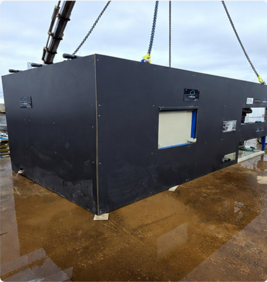
Craned onto the prepared pad
