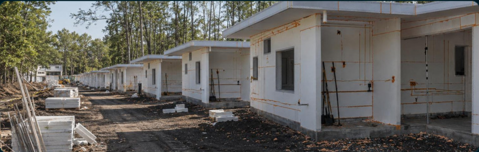
Panel-built housing under construction, envelope complete in days.
