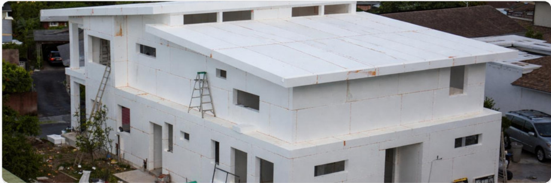
SABS structure, complete envelope before finishes.
